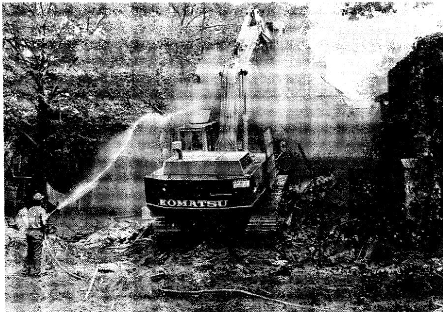
A bulldozer is used to demolish Roessler's gymnasium at High and Lewis streets in Perth Amboy
